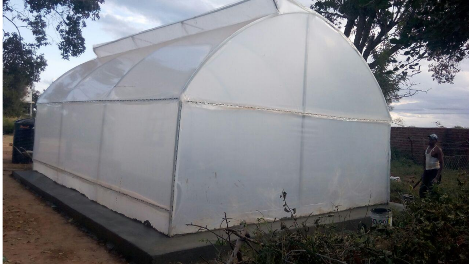
Green house solar dryer by QSM
