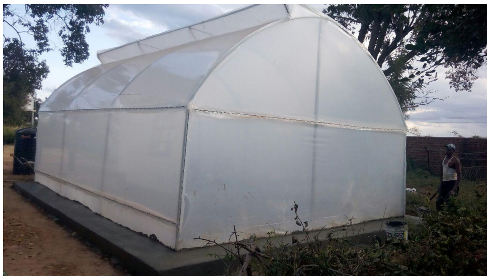
Dryer at RISE Group
