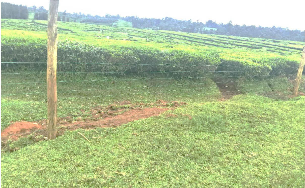
Photo 1: Completed and powered section of the electric fence
