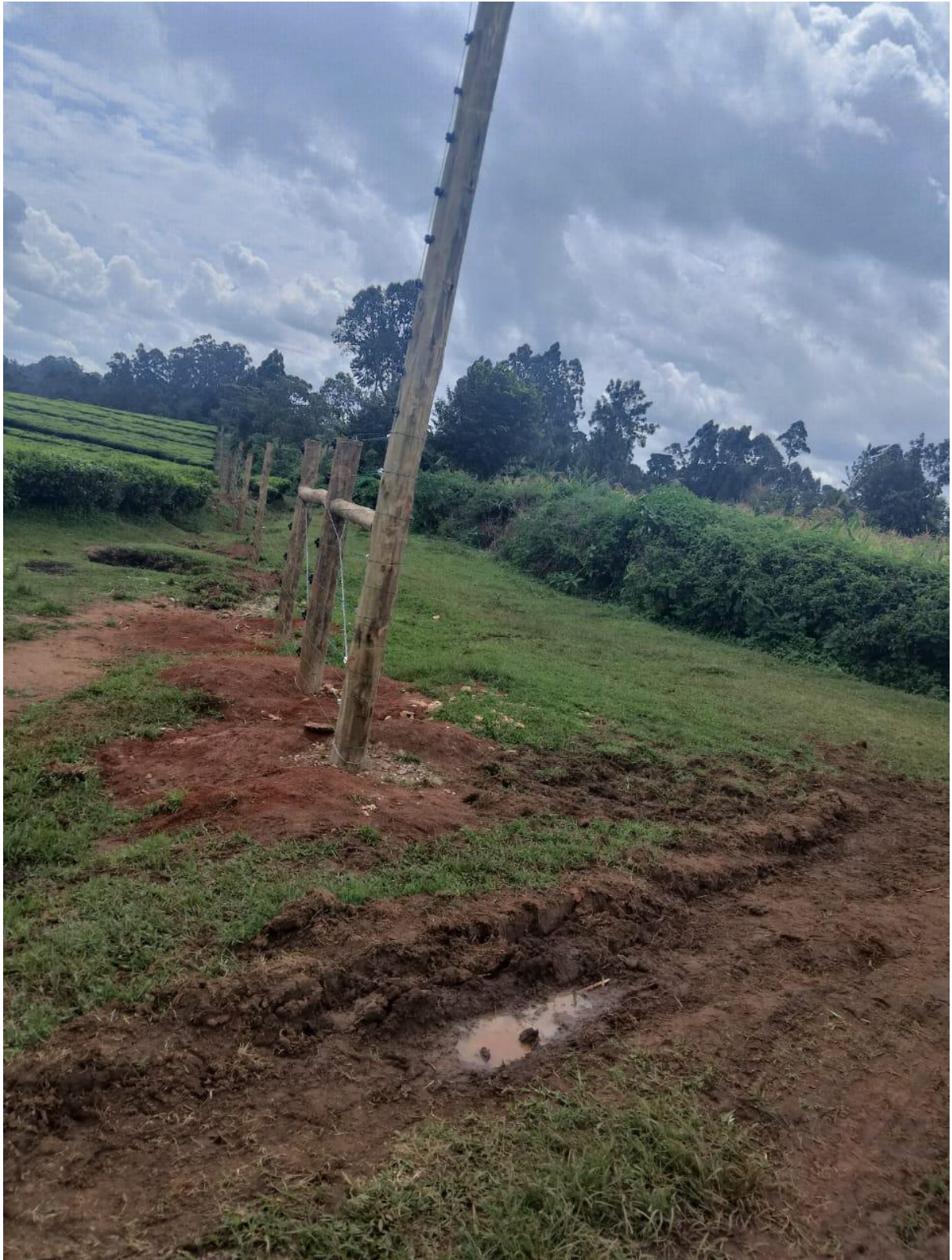
Photo 2: Ongoing section of the electric fencing
